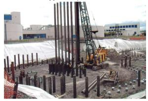
on 368 driven concrete filled piles. This proved to be the most efficient and economical solution, providing substantial savings and a much shorter schedule.
