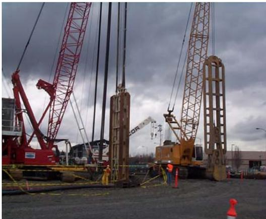
To overcome the verticality issue, the excavation equipment was equipped with real time verticality read-out equipment, which provided the field personnel data for a quick response.
