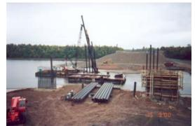
Two types of piling were used. At Piers 2 and 3, concreted-filled pipe piles went in. At Pier 1 and at the West abutment, however, these piles would likely have failed because of the clay consolidating under the embankment.
