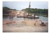
Instead, a pile-within-a-pile system was adopted: a combination of H-piles and pipe piles. The pipe pile went around each H-pile so the friction load from the clay caused by the embankment settling would be taken up by the pipe sleeves rather than by the H-piles. This design detail is commonly used in the Maritimes when high down drag loads are expected.
