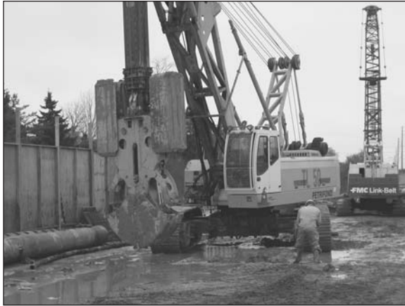
Figure 1. Slurry wall rig equipped with hydraulic clamshell
