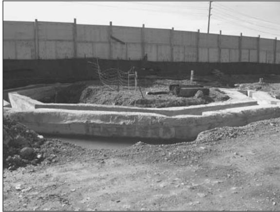
Figure 2. Guide walls at Access Shaft No. 3
