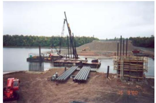
Two types of piling were used. At Piers 2 and 3, concreted-filled pipe piles went in. At Pier 1 and at the West abutment, however, these piles would likely have failed because of the clay consolidating under the embankment.
