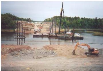
Instead, a pile-within-a-pile system was adopted: a combination of H-piles and pipe piles. The pipe pile went around each H-pile so the friction load from the clay caused by the embankment settling would be taken up by the pipe sleeves rather than by the H-piles. This design detail is commonly used in the Maritimes when high down drag loads are expected.
